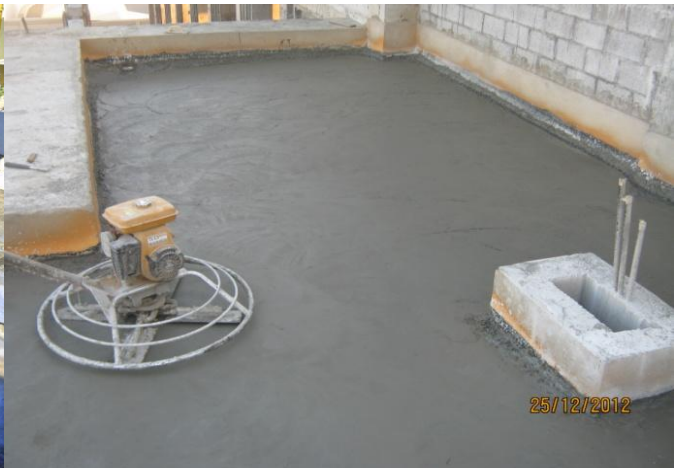
step #12: screed softening by the helicopter.
