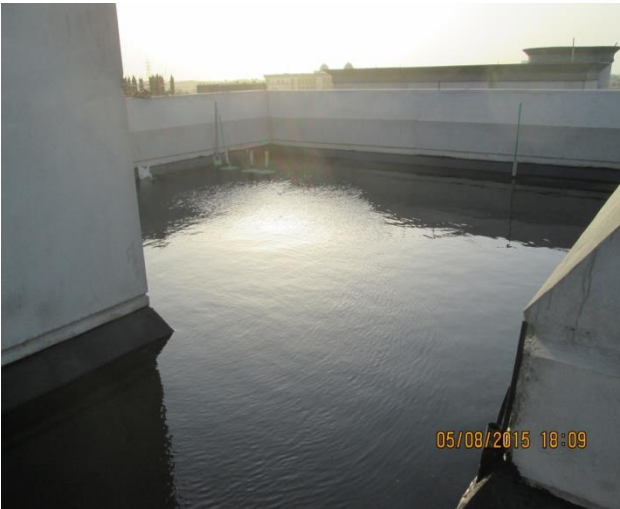
Step#9: Water testing..
