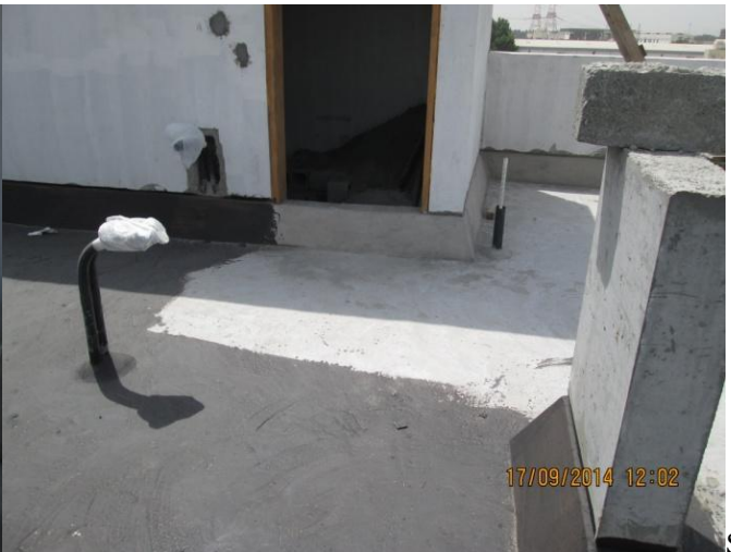
Step#4: Roof preparation, electrical conductors are well sealed
