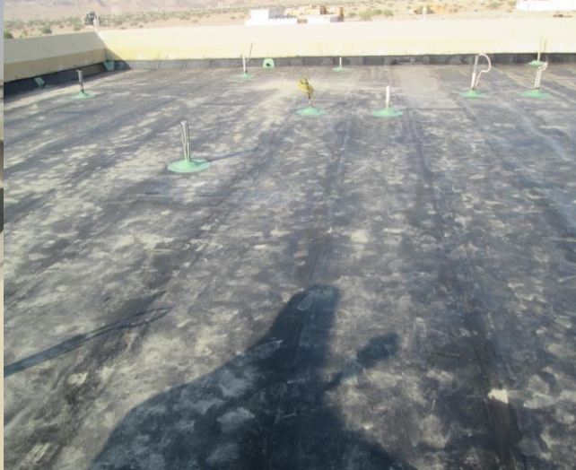
.Step#8: Install one layer APP elastomeric membrane.
