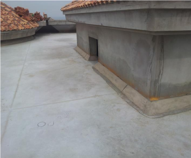
Step#9: expansion joints execution, SIZE: 20cmx20cm.
