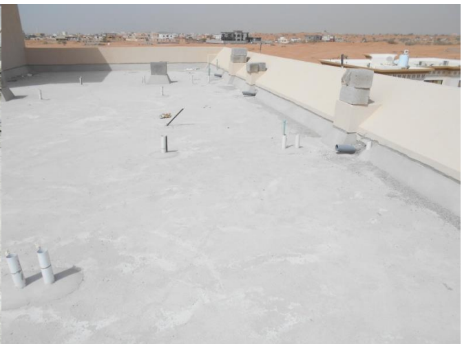
Step#6: 1.5x1.5 cm execution along the parapet.
