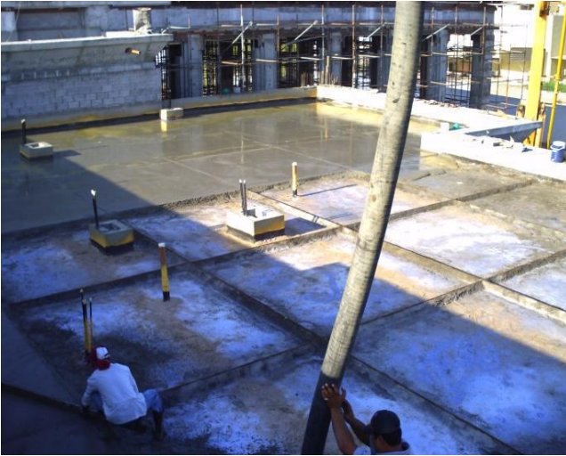
Step#7: screed casting.
