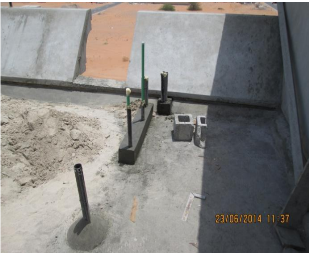
Step#3: Roof preparation, middle A/C pipes.
