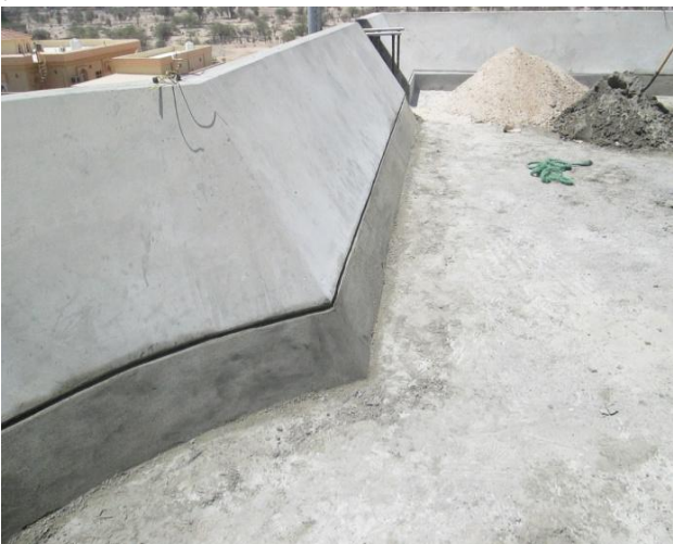
Step#5: slop corners 20x20 cm along with the parapet.
