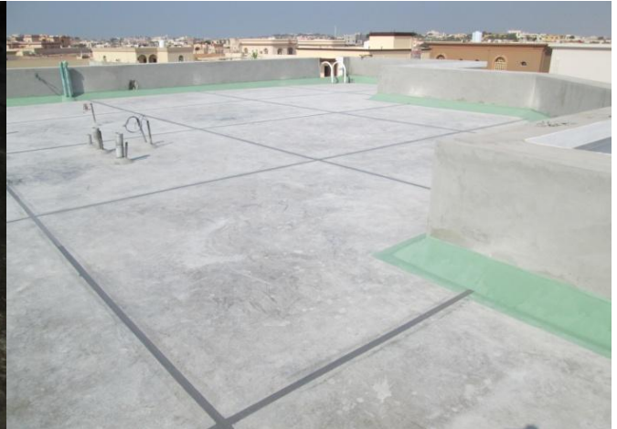
step#14: filling the expansion joints by: sponge then mastic.
