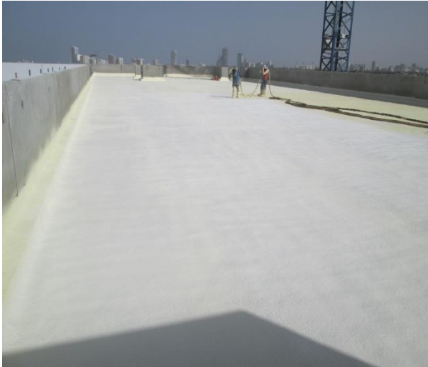
Step#2: polyurethane application.
