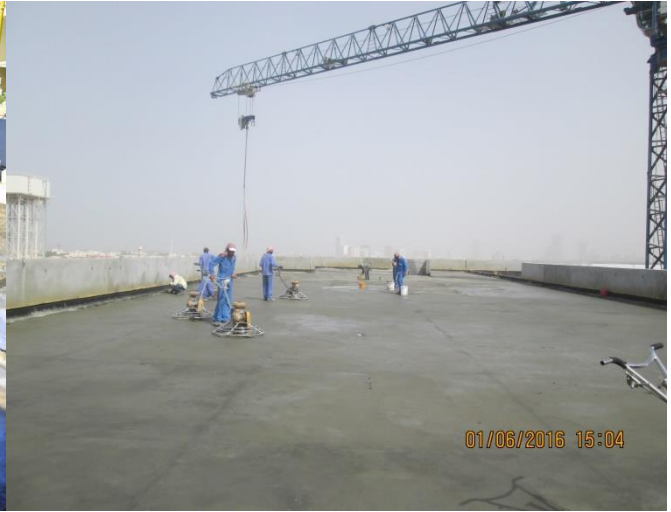
Step#8: screed softening by the helicopter.
