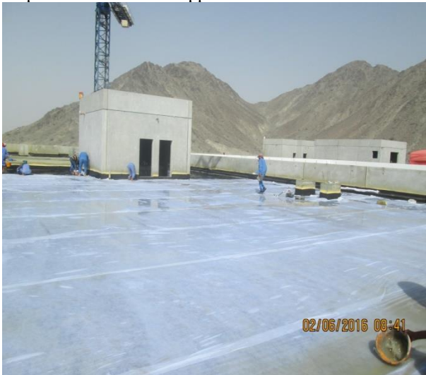
Step#5: Separation layers application.
