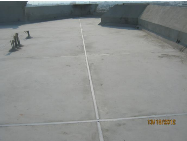
Step#11: filling the expansion joints by: sponge then mastic.
