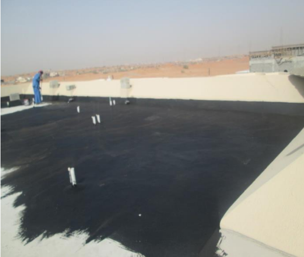
Step#7: applying cold bituminous primer
