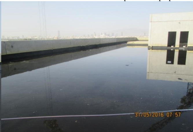
Step#4: Water testing.
