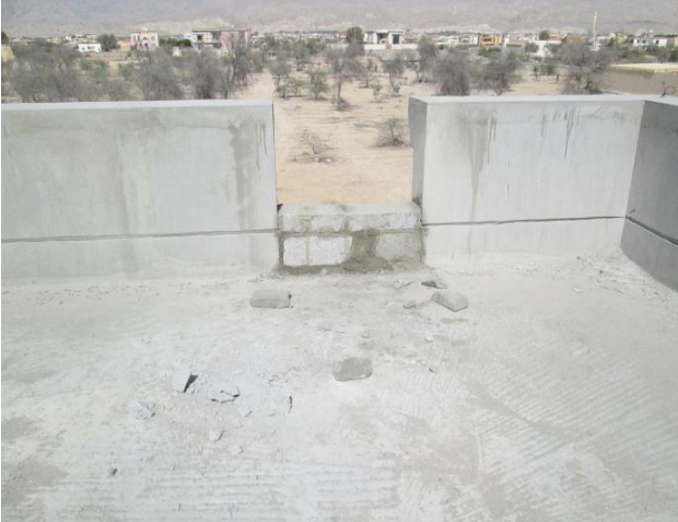
Step#1: Roof preparation, threshold placement.
