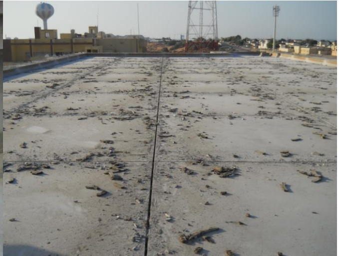
Step#10: Removing the flexible sheets.
