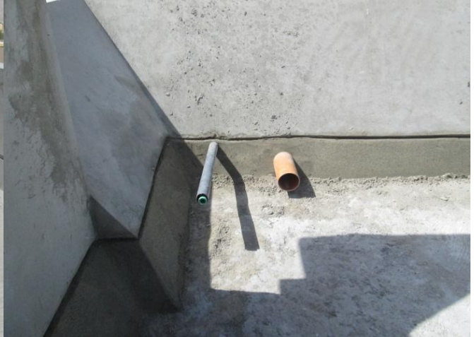
Step#2: Roof preparation, parapet A/C pipes.
