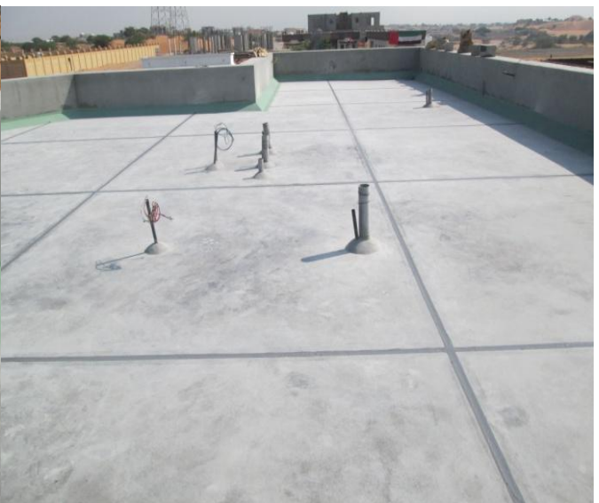
step#14: filling the expansion joints by: sponge then mastic.
