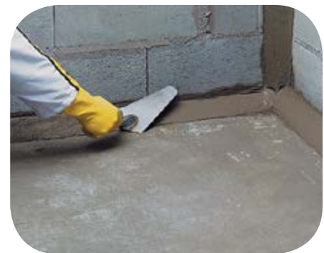
Corner chamfered with weberep 331 TX
